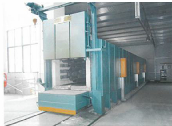
> 回火炉 / Stress relieving furnace
